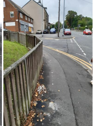
Swinnow Road Asbestos
