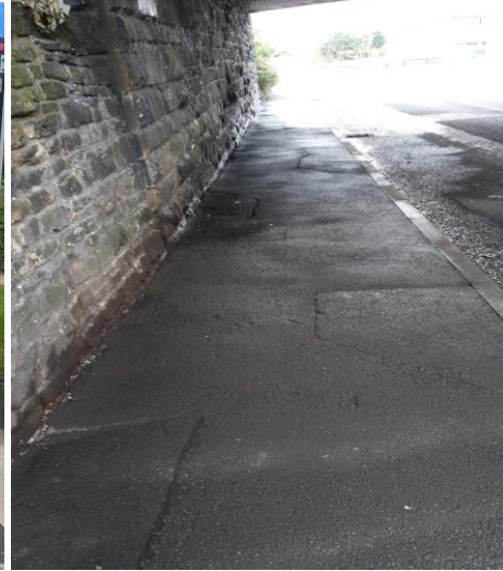
Amberley Rd Rail bridge clean-up
